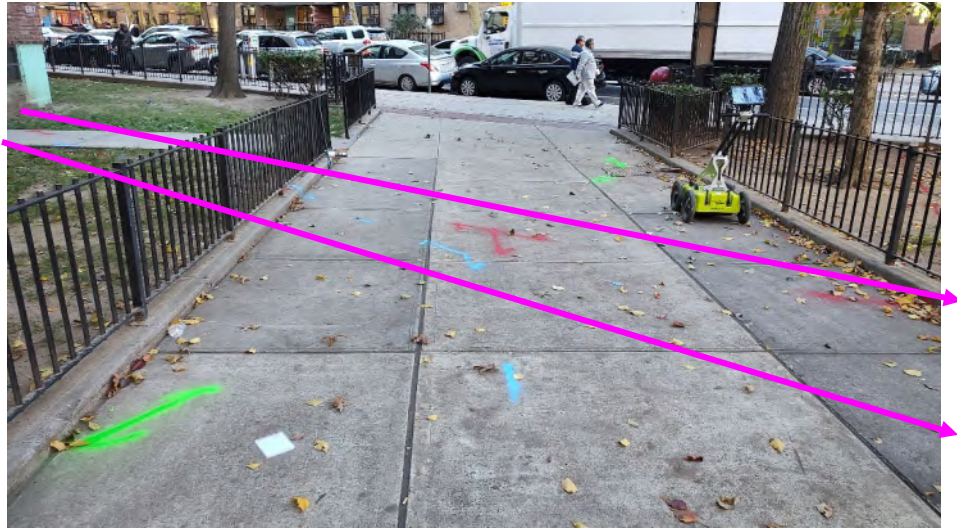
Photo 1 – Photo of the concrete walkway between Elliot 4 and the playground area. This area contained multiple utilities including storm drainage, electrical, and water lines. There was also a possible steam line leading from Elliot 4 towards Elliot 1, though this area was marked out later in pink as a trench to avoid during drilling activities.
